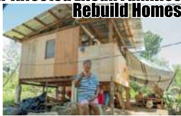
Through the support of the Aboitiz Foundation, displaced Liloan residents like Adela Gales are rebuilding their homes for a fresh start
