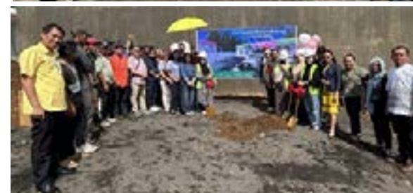
CARD MRI staff, management, clients and partners took part in the groundbreaking of the CARD Care Clinic facilities in Marawi City (left) and Cotabato City (right), marking a significant move toward bringing accessible primary healthcare to the communities.
