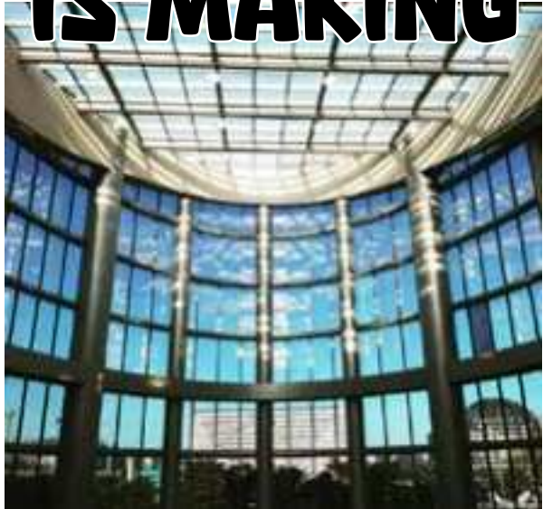
Natural light streams through the skylights of SM Supermalls, helping reduce electricity consumption while creating a bright, welcoming space.
