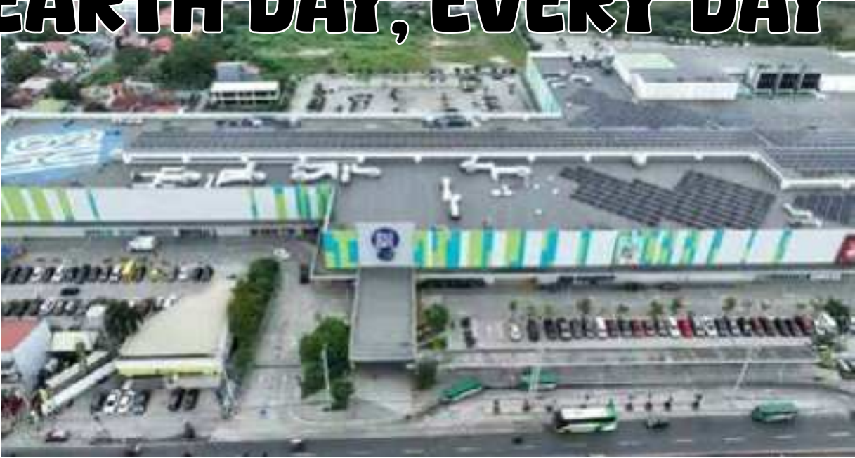
SM City Tanza powers up with 2,286 solar panels, generating a peak capacity of 1,257.30 kW—part of SM
