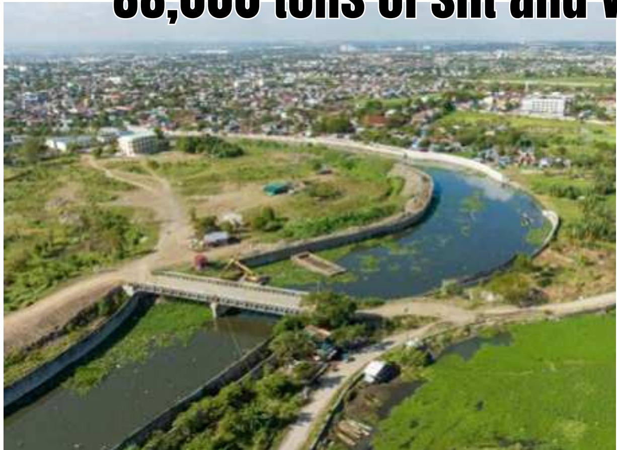
A total of 87,899 tons of silt and solid waste have been removed from 3.2 kilometers of Biñan River, restoring the depth, width and natural flow of this waterway draining out to Laguna Lake.
