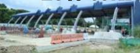
Governor's Drive Toll Plaza Construction progress
