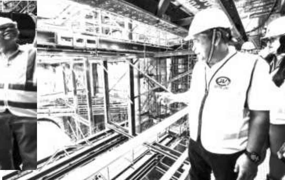
Department of Transportation Secretary Jaime Bautista visits the site of the ongoing construction of the Metro Manila Subway Project at the North Ave. Station on March 7, 2024. (PNA photo by Joan Bondoc)
