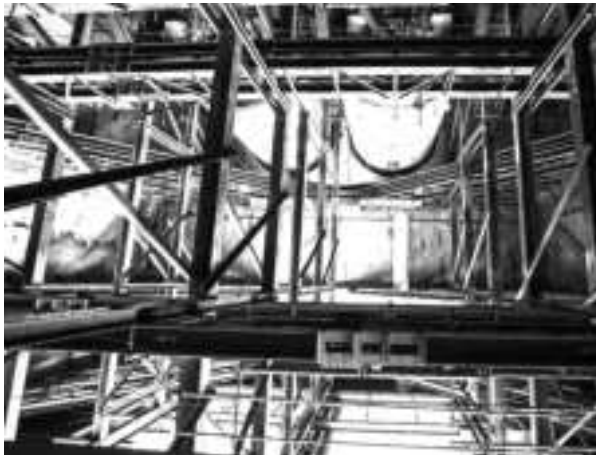
The tunnel boring machine at the Metro Manila Subway Project's North Avenue Station (PNA photo by Joan Bondoc)
